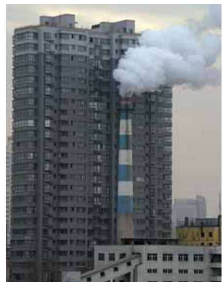
Anticipating the demolition of a power plant, the construction of a new block of flats has already started...and finished.
