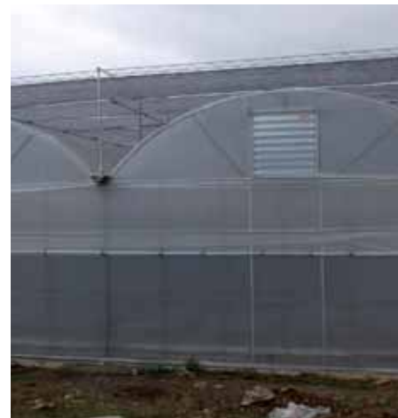
Exterior of the demonstration greenhouse: double plastic film and an inner and outer protection screen.
