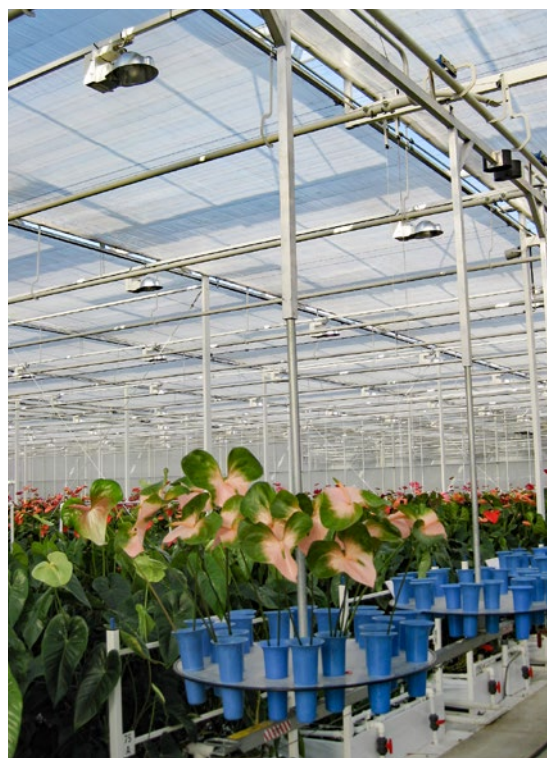
Hanging harvesting system in combination with the upper net of the heating
