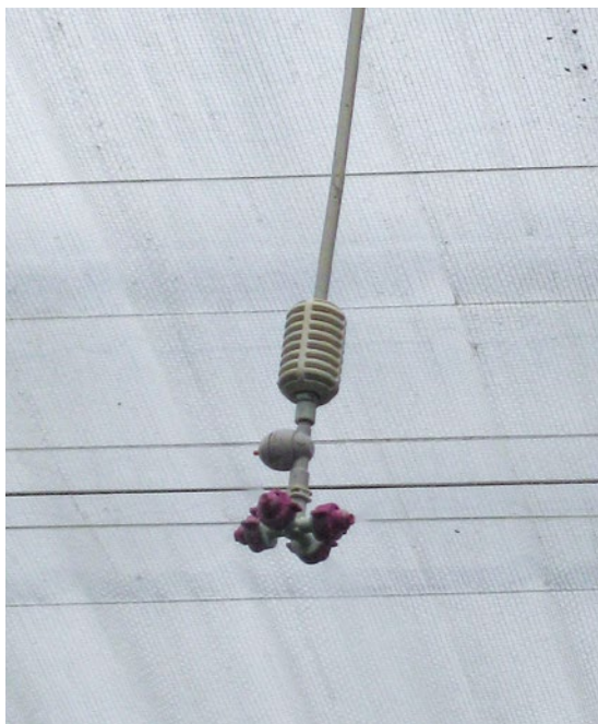
Simple low-pressure humidification
