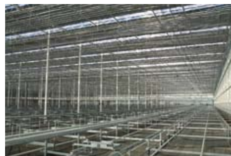
The diafragmascreen® of Anthura's new construction project
