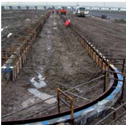
The foundation is under construction
