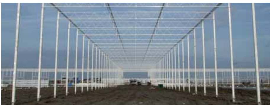
Steel skeleton of the greenhouse
